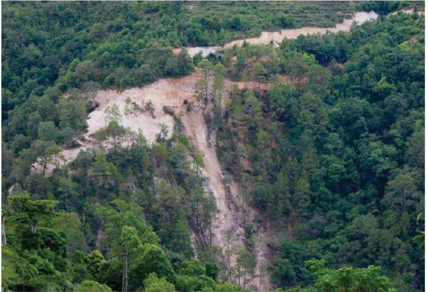
Figure 2.2. Landslide following road construction in Bhutan
